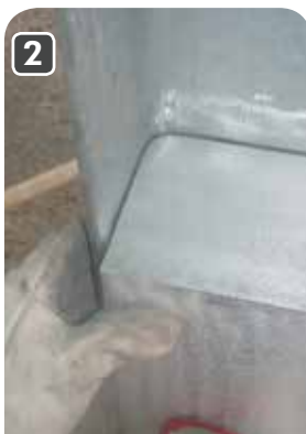
2 Metal inserts preparation
